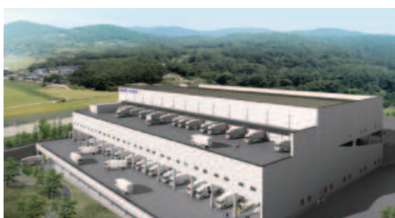
DPL Anpyeong Logistics Center
